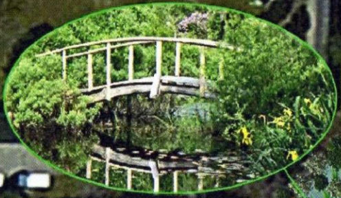
Scenic bridge crossing to wildlife viewing platform
